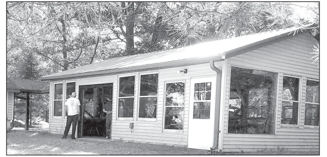
Installing the screens.
