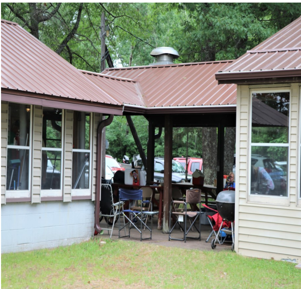
New metal roof on all of the buildings
